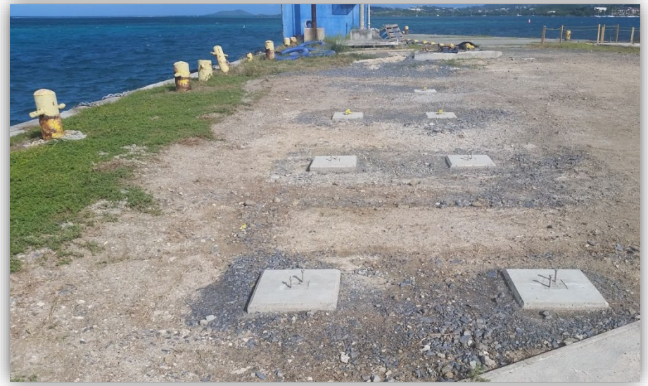
Jetty area pipe support foundation
