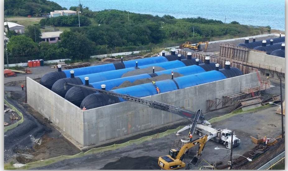
South mound being backfilled with crushed stone
