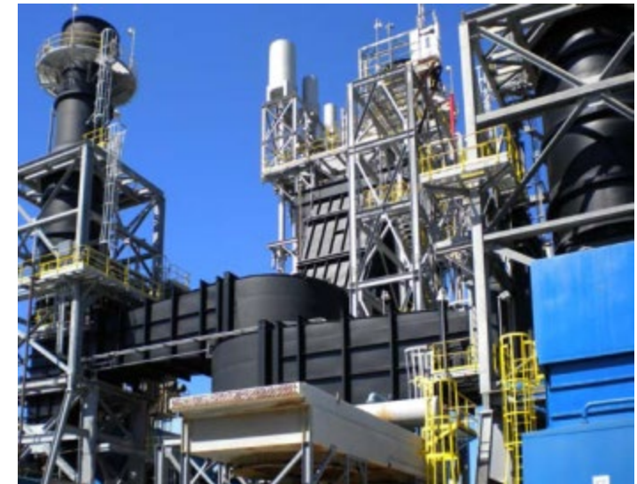
Heat Recovery Steam Generator (St. Croix)
