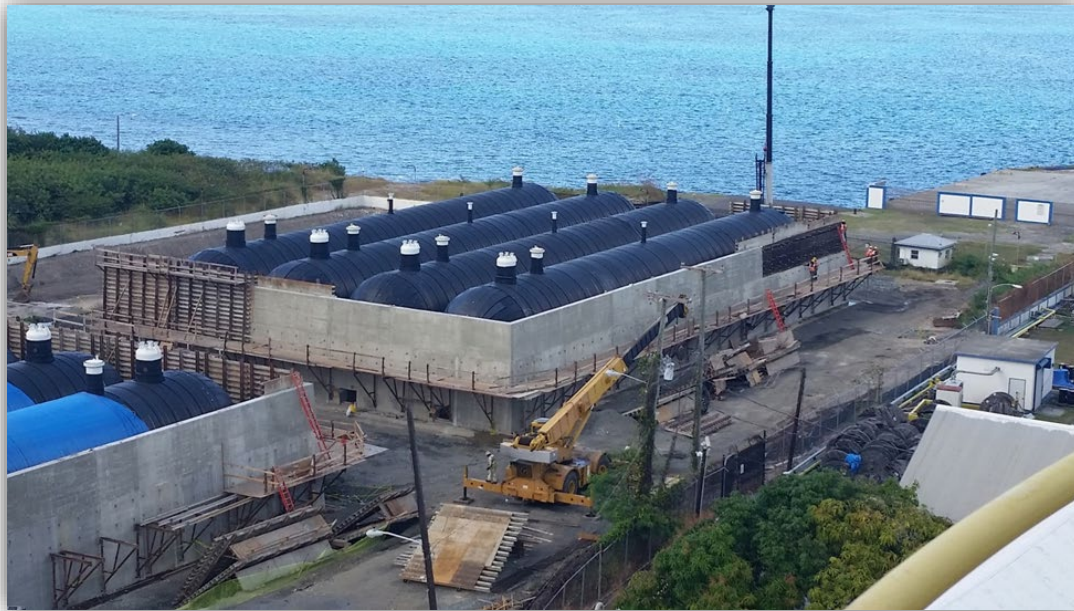
North mound top wall forms and rebar
