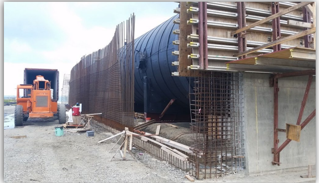
North mound west wall rebar installation
