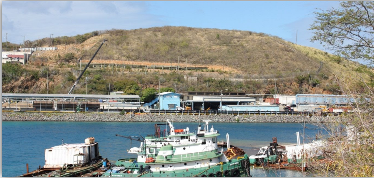
Project site prior to blasting and construction activity
