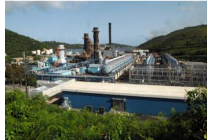
Randolph E. Harley Generating Substation (St. Thomas)
