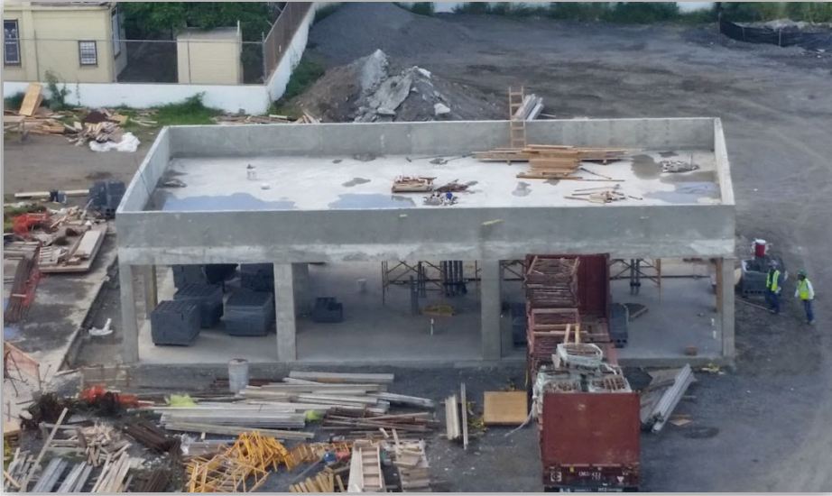
Vaporizer area – boilers set on slab, pipe supports, excavation for flare foundation
