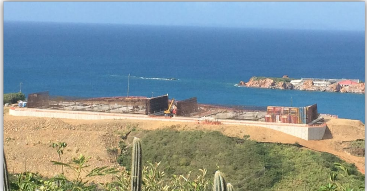
Current project site
