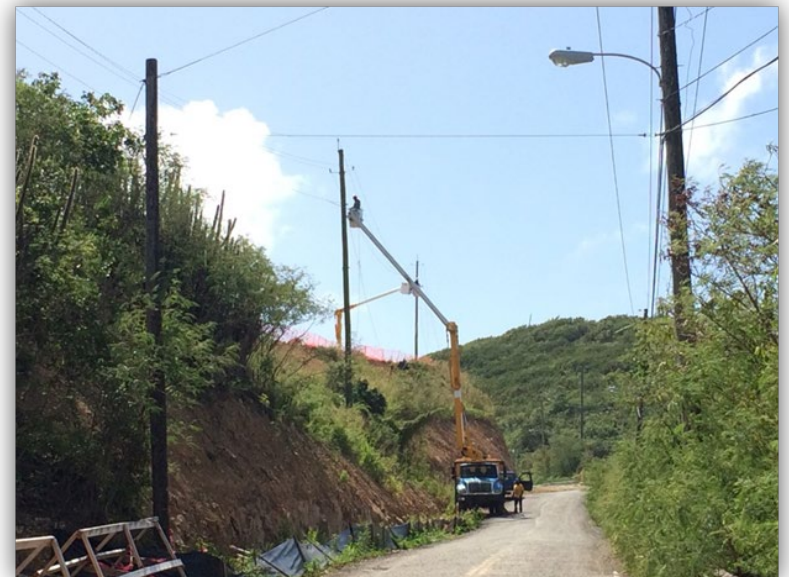
Raising utility lines for LPG tanks transport
