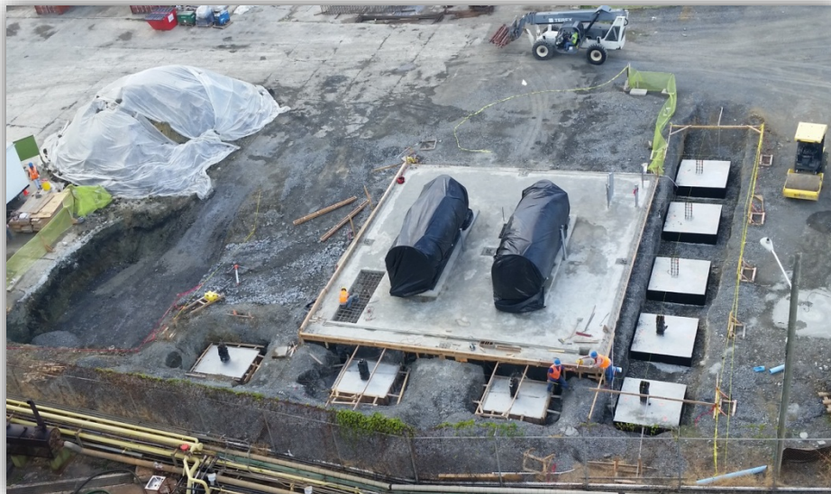
Vaporizer area – boilers set on slab, pipe supports, excavation for flare foundation
